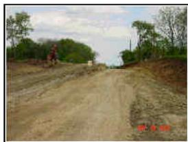
As this article is written on June 22nd, the original highway surface is gone, and the roadbed has a wide, thick, coarse gravel base. No concrete has as yet been poured.
